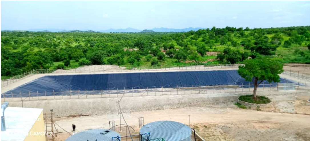
Completed TSF with fencing
