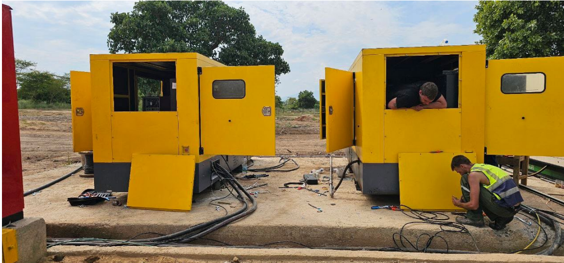
Commissioning of generators on site
